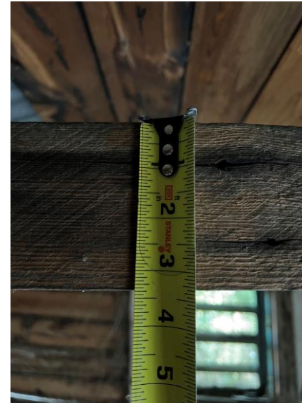
Roof joist dimensions
